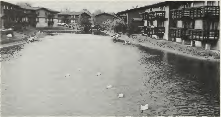
Developer of apartment complex above in Indianapolis used an excavated area for storm water storage, recreation, and for scenic value. Storm water is routed into this area and released through an outlet at a retarded rate. Right, improper disposal of surface water caused gully threatening a home in Des Moines. Below, sediment and debris fill channel of small stream where it passes through a development in Washington State.
